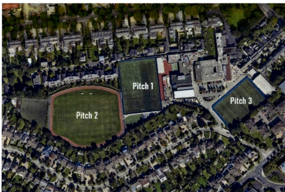
Figure 3 – Overview of pitches where lighting is to be installed
